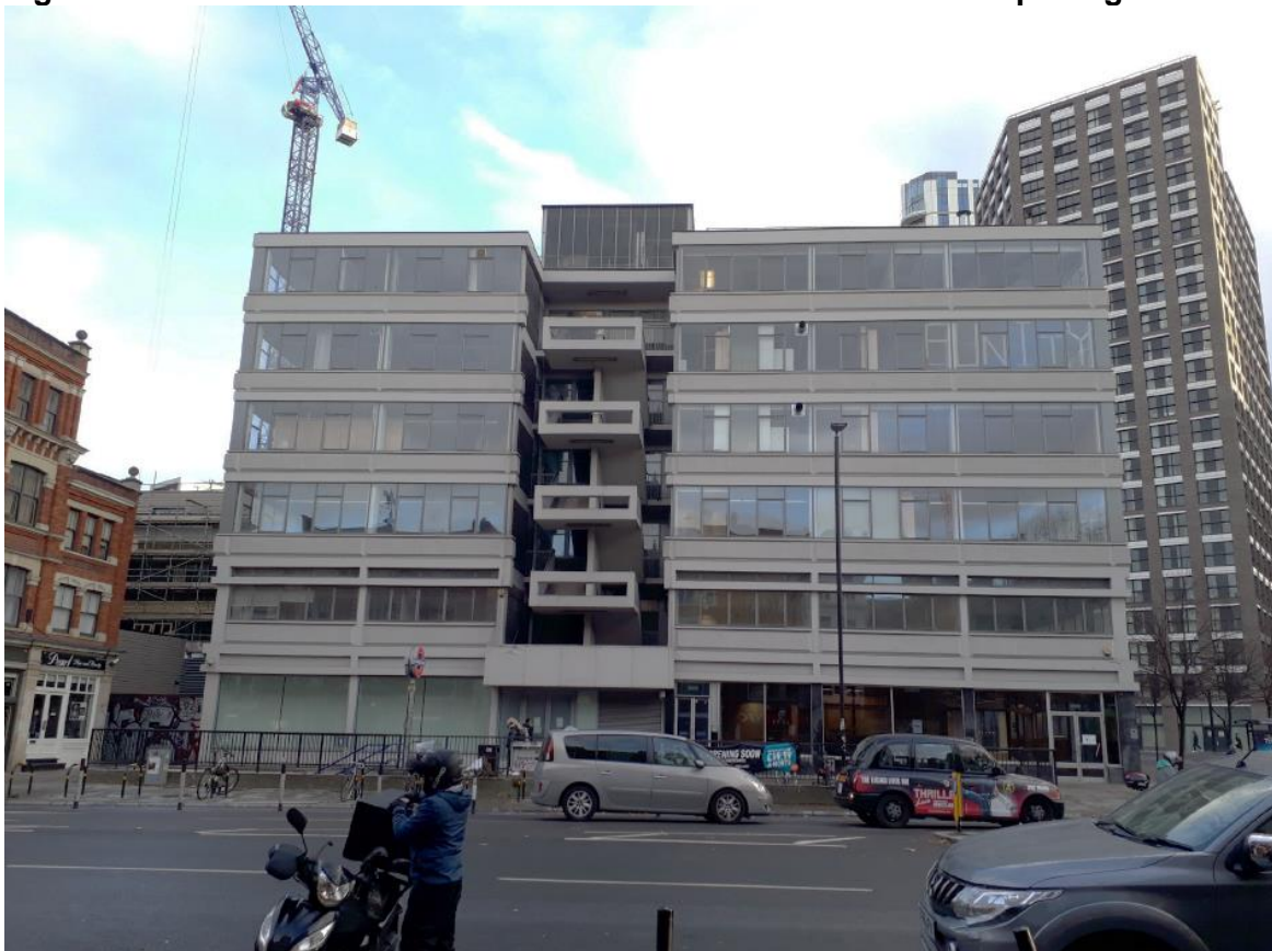
Figure B View of north elevation
