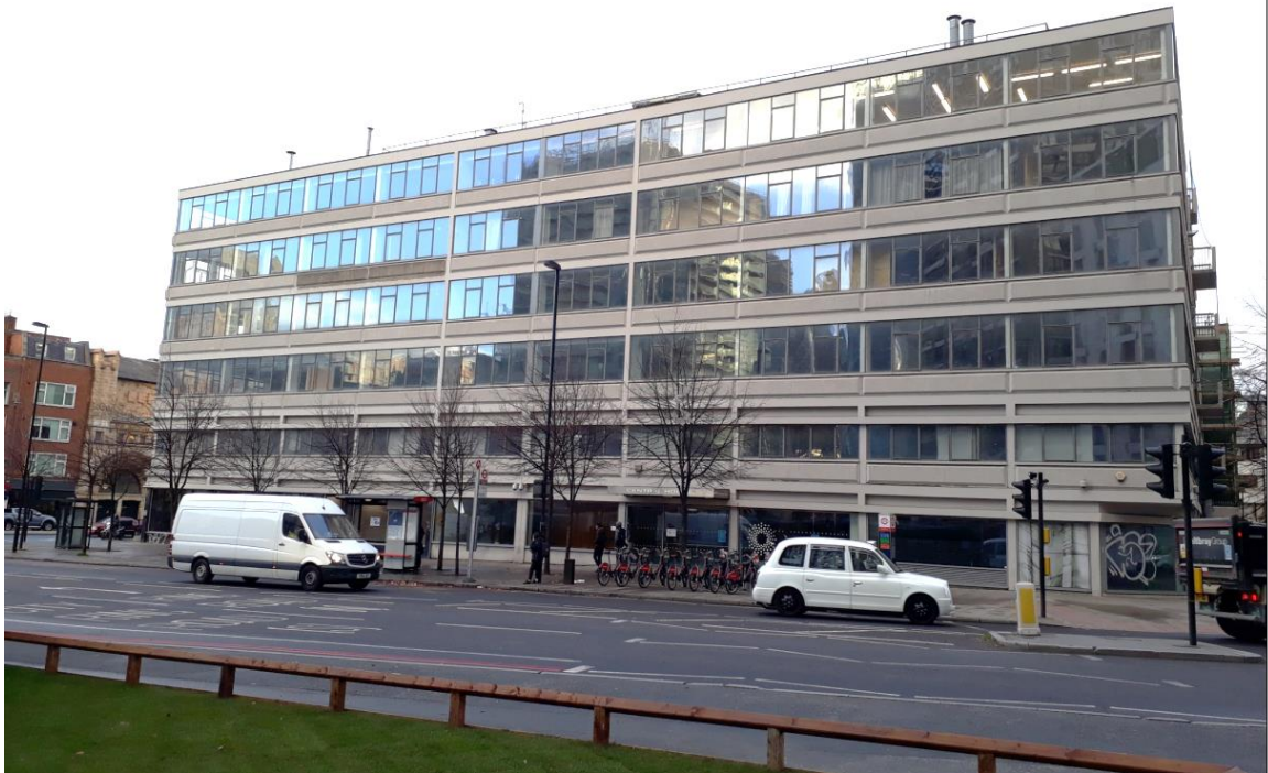
Figure C View of west elevation (above)
