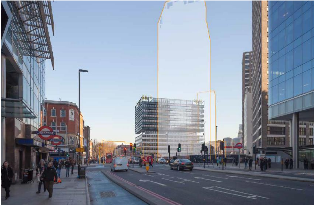
Figure 7: Verified view of scheme with Whitechapel High Street Conservation Area in background and consented context (2 Whitechapel High Street to left with Aldgate Place Block B in foreground and 27 Commercial Road to the right)
