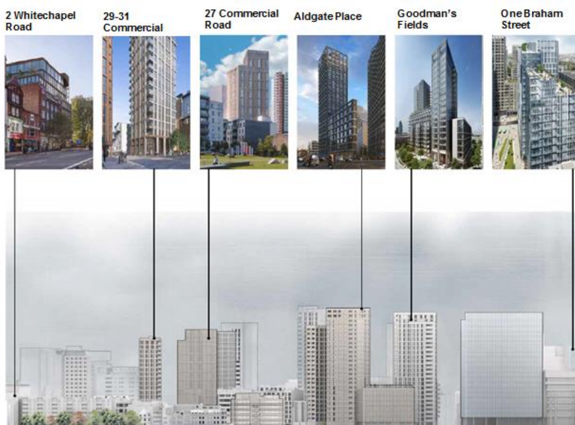
Figure 2: Existing building in its emerging tall building context
