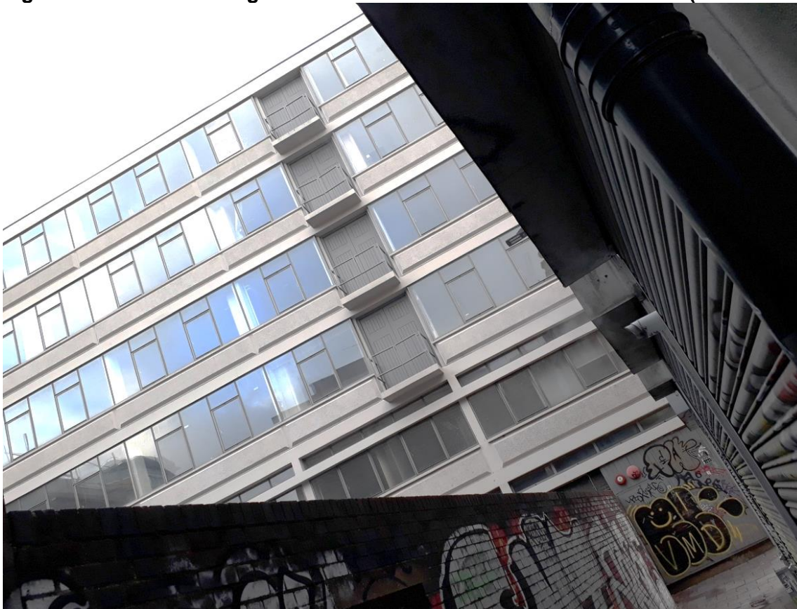
Figure F View of east elevation from White Church Passage
