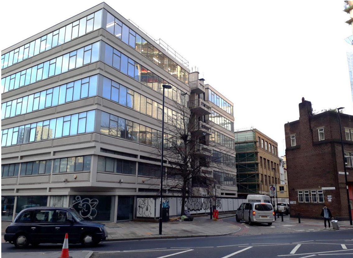
Figure E View of Manningtree Street elevation from Commercial Road(Above
